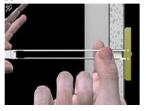
Hold the ends of straps between thumb and forefinger and pull toward you until channel rests flush behind wall. Slide plastic cap along straps with other hand until flange of cap is flush with the wall.
