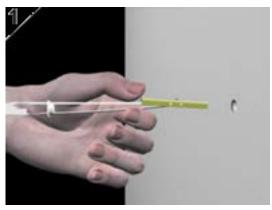
Drill a ½" hole. Hold the metal channel flat alongside plastic straps and slide channel through the metal channel through the hole. The minimum clearance behind the wall is 1 7/8".
