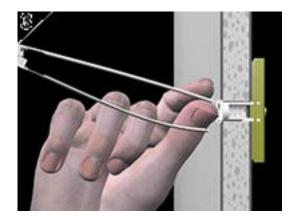
Snap straps at wall by pushing side to side snapping off straps level with flange cap.
